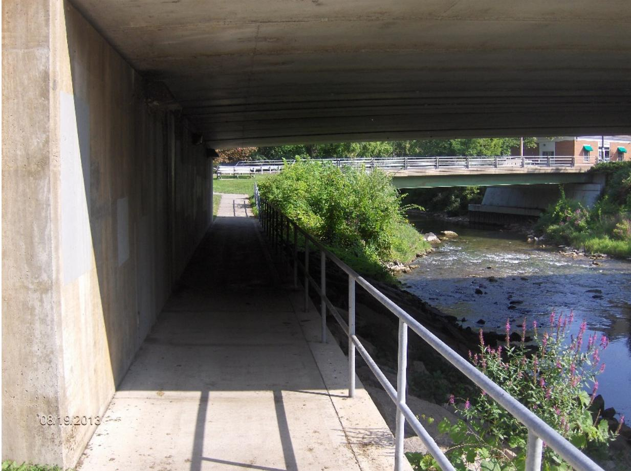
Permits would be required from NYSDOT, NYSDEC, and USACoE. Construction would include the placement of large stones under the highways at the creek's edge along the eastern most wall of the two box tunnels and placing a concrete slab on top forming the trail. Amenities would include LED solar lighting, safety railing, signage, and trail connections including contour earth moving, filter fabric, crushed limestone (crusher run/runner crush), and stone dust for about 800 linear feet of trail.
